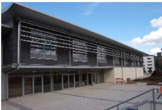
The conference venue, R Block building, at Frenchay Campus of UWE, includes many innovative sustainable design features.
